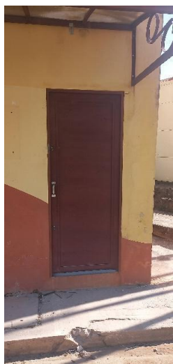
FIG 23 - Porta Frontal Datacenter
